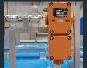
▲ Gas leakage alarm unit
